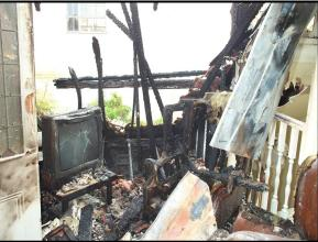
It was apparent that the heater had been placed very close to the edge of the couch which had ignited. The fire then spread through the ground and upper floors. Analysis of the couch was carried out for the presence of an accelerant, but this proved inconclusive.
