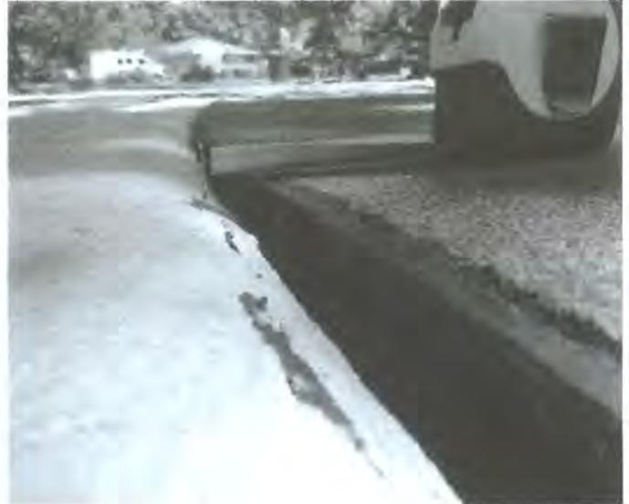
Over time, the unitary surface may separate at the seams or from the border creating gaps, openings or changes in level that will require repair.
