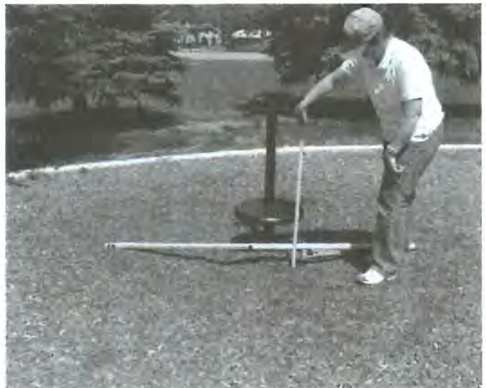
Loose fill materials, like EWF, may experience undulation of the surface material and or displacement under heavy use areas with motion such as at swings, slides, sliding pools, climbers, spinners and teeter totters. This will require the surface material to be raked level, filled and compacted so that the clear ground space is level in all directions for a safe transfer onto and off the equipment.
