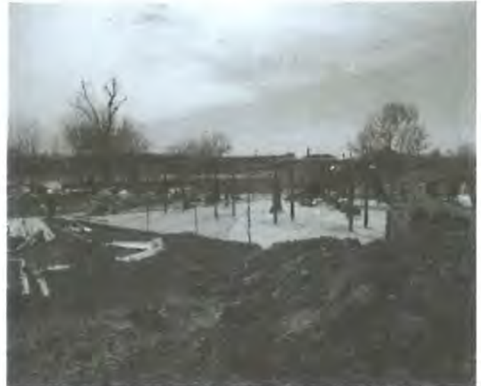
The playground site has been graded with earth-moving equipment. The concrete base has been prepared and is awaiting the application of the poured-in-place rubber (PIP) system. At this site, the playground equipment and surface system will be installed by a contractor specializing in playground construction.
