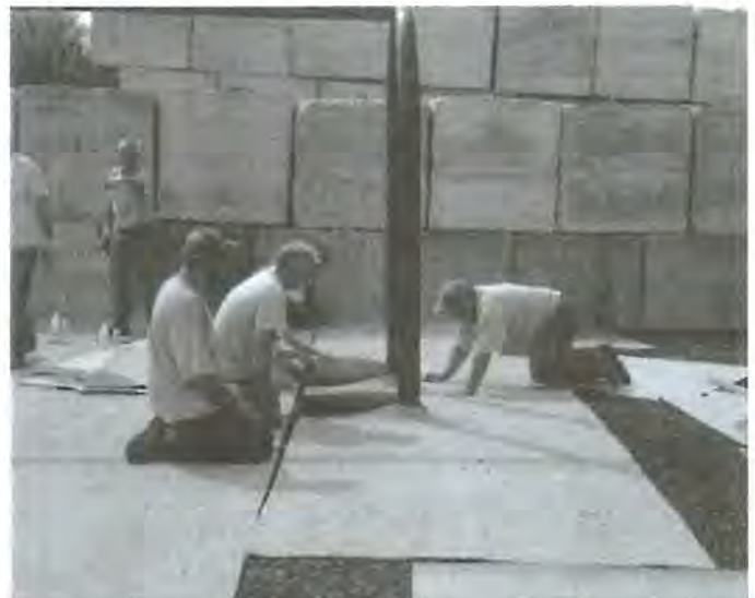
The base layer of crumb rubber has been installed. The top layer, a rubber mat system, is fit around equipment and the seams are joined. Both the equipment and surface system at this site will be installed by the park maintenance crew.
