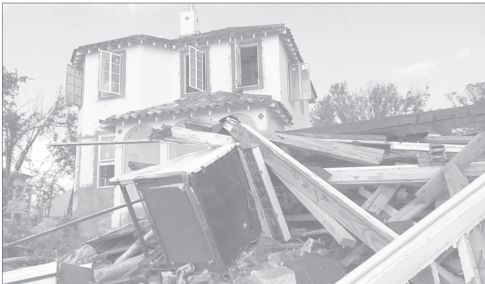
Above: In this photograph taken from video, a beach home in Bay St. Louis, Mississippi is in the rebuilding process, Aug. 18, 2006. The Gulf Coast in southern Mississippi is still reeling from the effects of Hurricane Katrina a year later. Below: A tattered American flag flies over the Barousse's home in the Irish Bayou neighborhood of New Orleans, Louisiana, Aug. 1, 2006. "Most of these people are not coming back," Gene Barousse says. Of the 80 to 90 families in the almost-rural community of the Irish Bayou section of New Orleans, 12 remain, he says.
