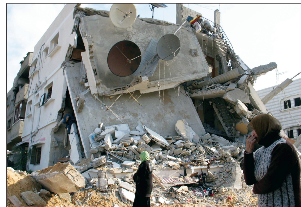
Maha al Sultan, right, surveys the damage to her family's home in Gaza City; the building housed six families and 55 people, all of whom survived by fleeing to a relative's house when Israeli tanks moved in.
