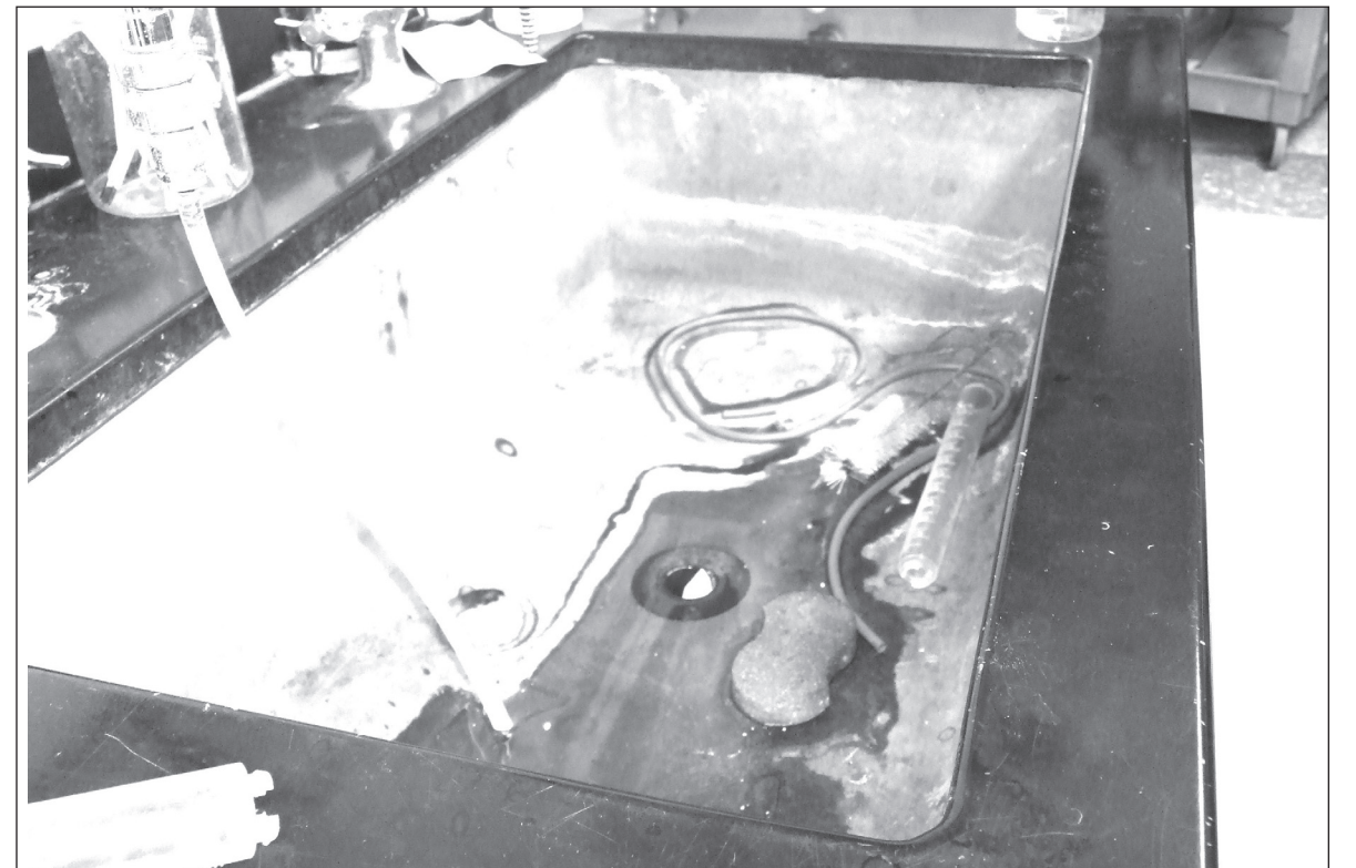
Above: a sink in the science lab that is rusting and is in dire need of replacement before further contamination occurs and
