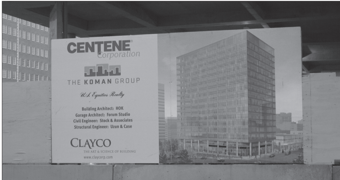
The sign around the construction site shows a projection of what the Centene building will look like once finished. The builders plan to make the new Centene headquarters 17 stories.
