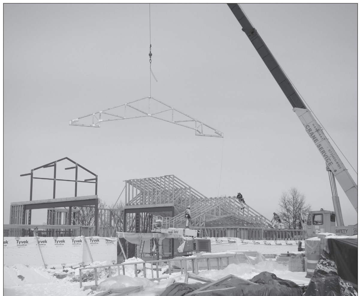
Ongoing construction work in the St. Louis area is being funded by money appropriated to the city from the federal stimulus package that went into effect in 2009.
