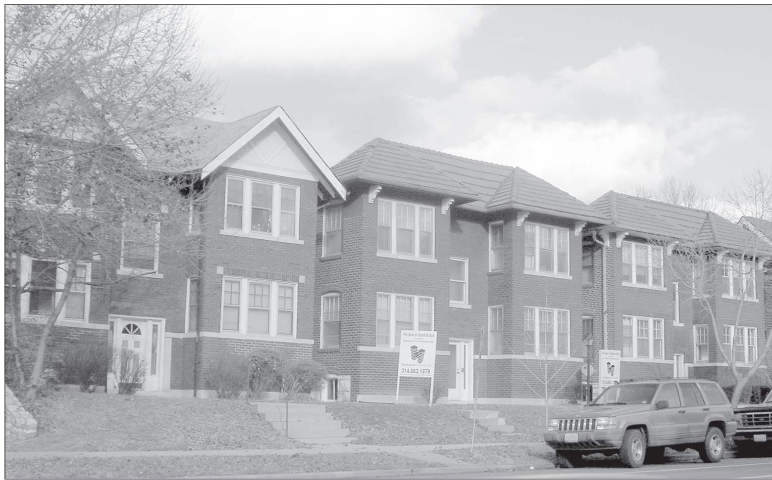
PROPERTIES ON CLAYTON Road which have caused controversy among residents in the Demun Area. After two years and numerous public hearings, the city has developed an Urban Design District in order to set a specific plan and ease controversy in the area.
