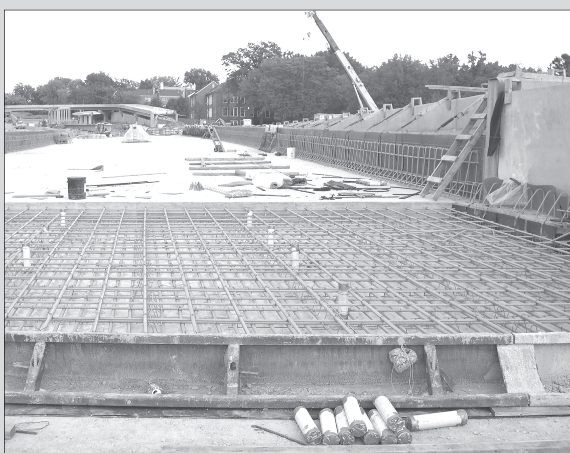
FOUNDATIONS FOR THE St. Louis County MetroLink extension are laid out across Brentwood Blvd and along Meramec Elementary. Despite some worry about noise and traffic, the majority of St. Louis residents are eagerly anticipating the new transportation system, which will extend west throughout St. Louis County.
